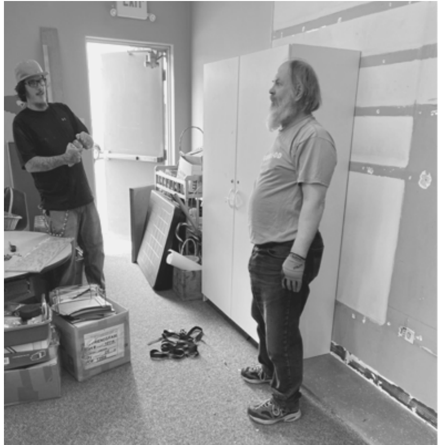
Mike Bender and Cliff Thompson removing cabinets
